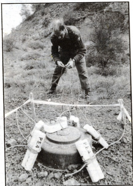
Working alone the Eng Off prepares the detonator and safety fuse.
